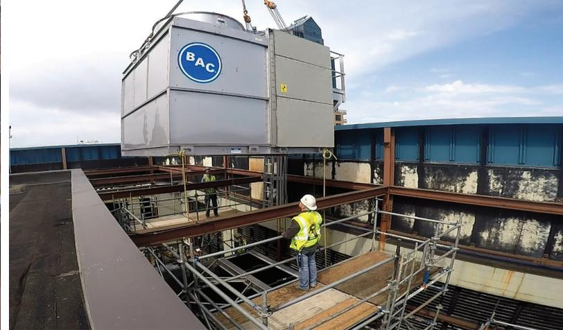
Left: Installed cooling tower // Middle: Lifting cooling tower with Vic’s crane // Right: Placing cooling system on Galtier roof
